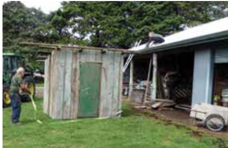
John Little's shed for 'The Glen.' Silja cleaning shed spouting
