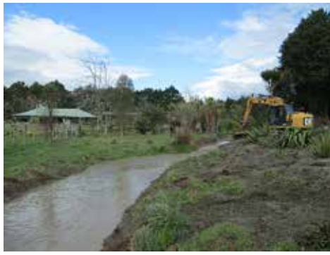
Digger removing soil and vegetation before heavy rains. Lucky! September 2018.
