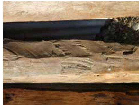
Dairy shed posts. Sound. Clear axe marks. 120 years old and to be recycled.
