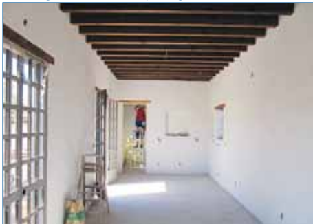
25. Office building getting finishing touches. Oregon beams and high ceiling will keep the room cool.
