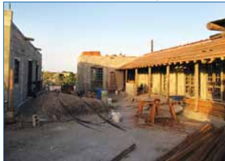
26. Alastair's home. Built in a traditional Mexican style with a tile roof, brick cladding and plastered stucco walls. 6m
