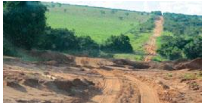
Weaving along 70 kms of road was bad enough but it was repeated, three days later. Mato Grosso do Sul
