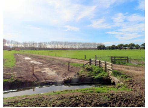
Overflow causeway. This will ensure any future cyclones can't flood the homestead
