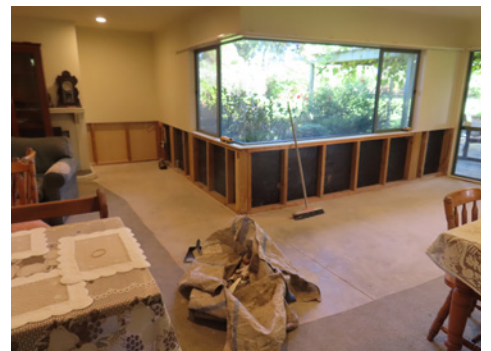
Carpets lifted, underlay silt laden. Curtains ruined 18 February 2023
